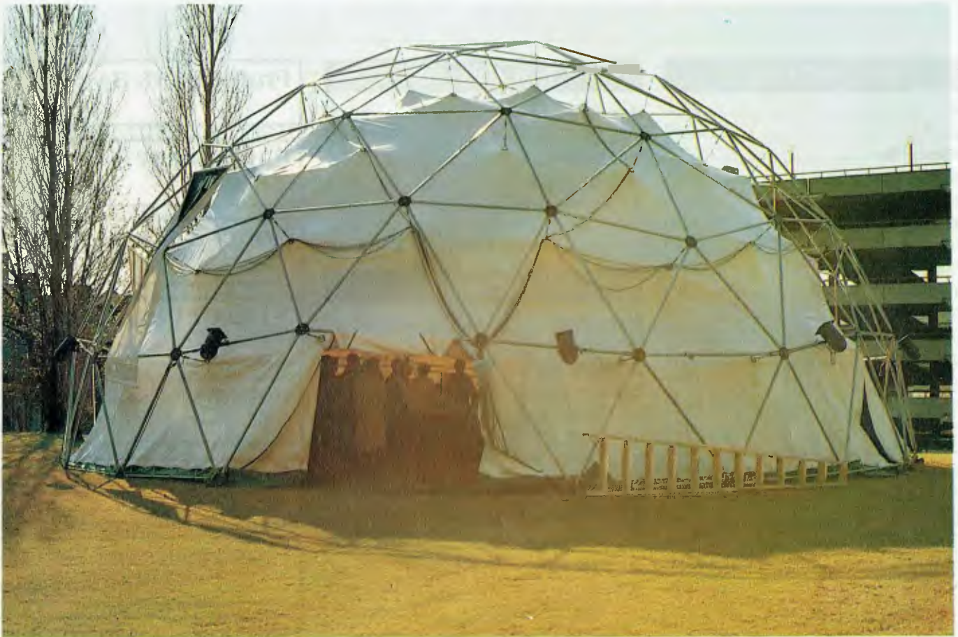
The geodesic dome on the lawns of the Seymour Centre. The dome was chosen for portability, strength, and its shape, which is well suited to three dimensional sound.
